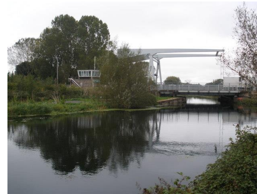
Hinged lifting bridge
