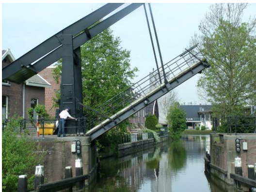
Hinged lifting bridge
