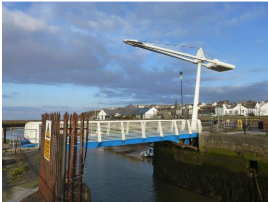
Hinged lifting bridge
