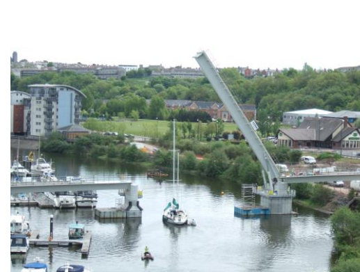
Hinged lifting bridge
