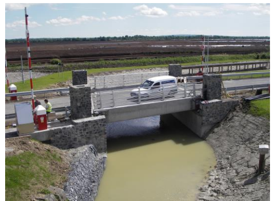
Vertical lifting bridge
